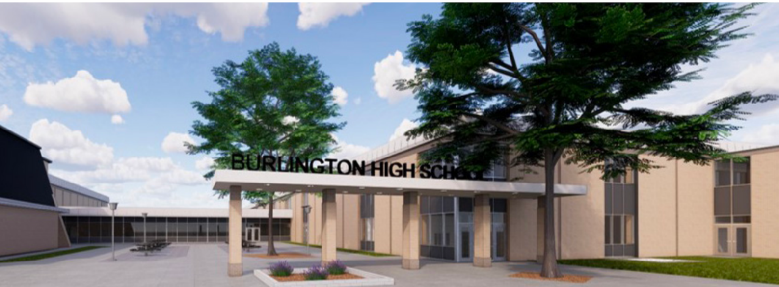
BURLINGTON HIGH SCHOOL MAIN ENTRANCE
